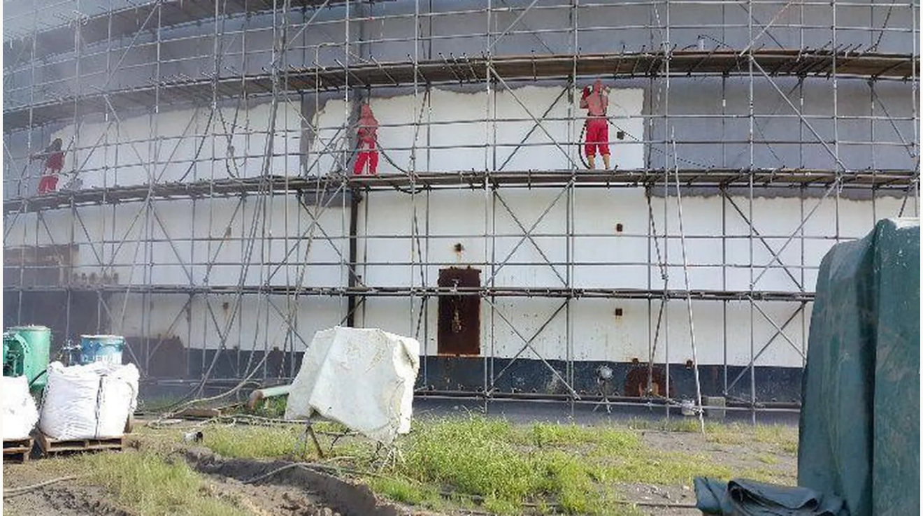
STORAGE TANK REHABILITATION AND COATING, ESCRAVOS TERMINAL
